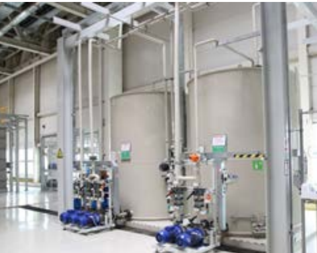
Our pretreatment water reuse system reduces water consumption and wastewater discharge.
