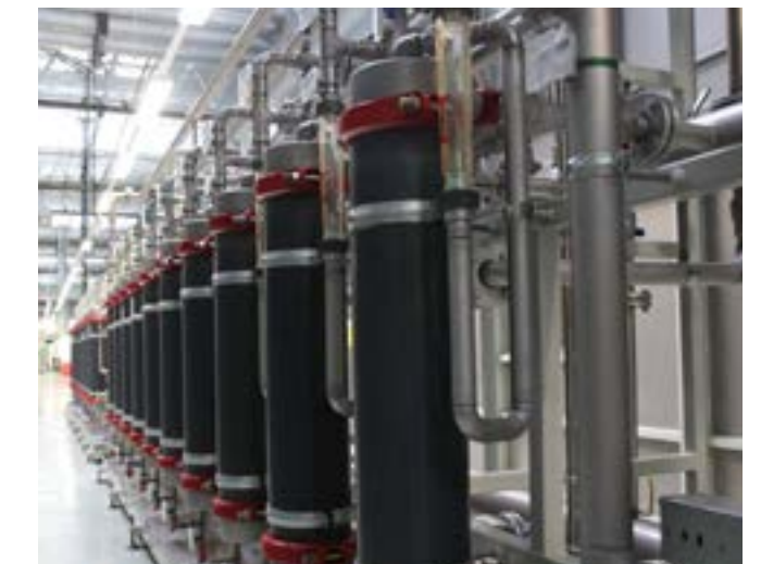
Our electrocoating ultrafilter system reduces wastewater discharge.
