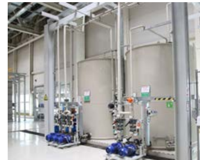
Our pretreatment water reuse system reduces water consumption and wastewater discharge.
